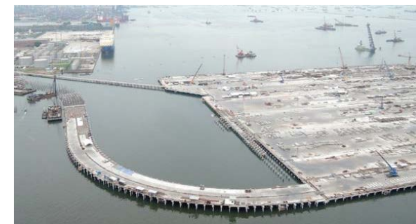
New Tanjung Priok Port Project 1
